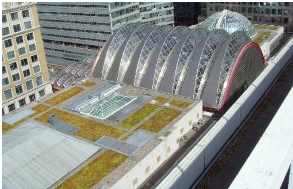
Green roofs at Canary Wharf (John Archer)
