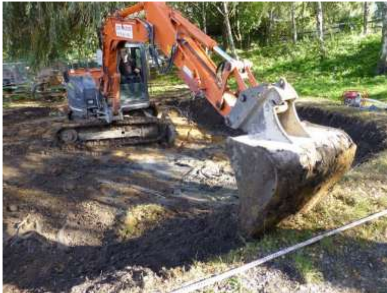
Digging a new pond at Mudchute (John Archer)
