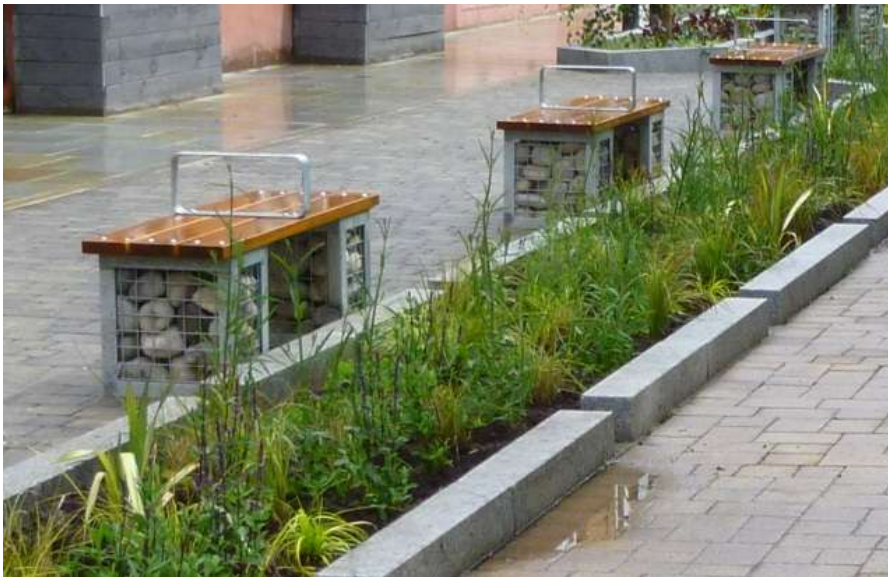
Gabion benches provide habitat for invertebrates (Jessica Bastock)
