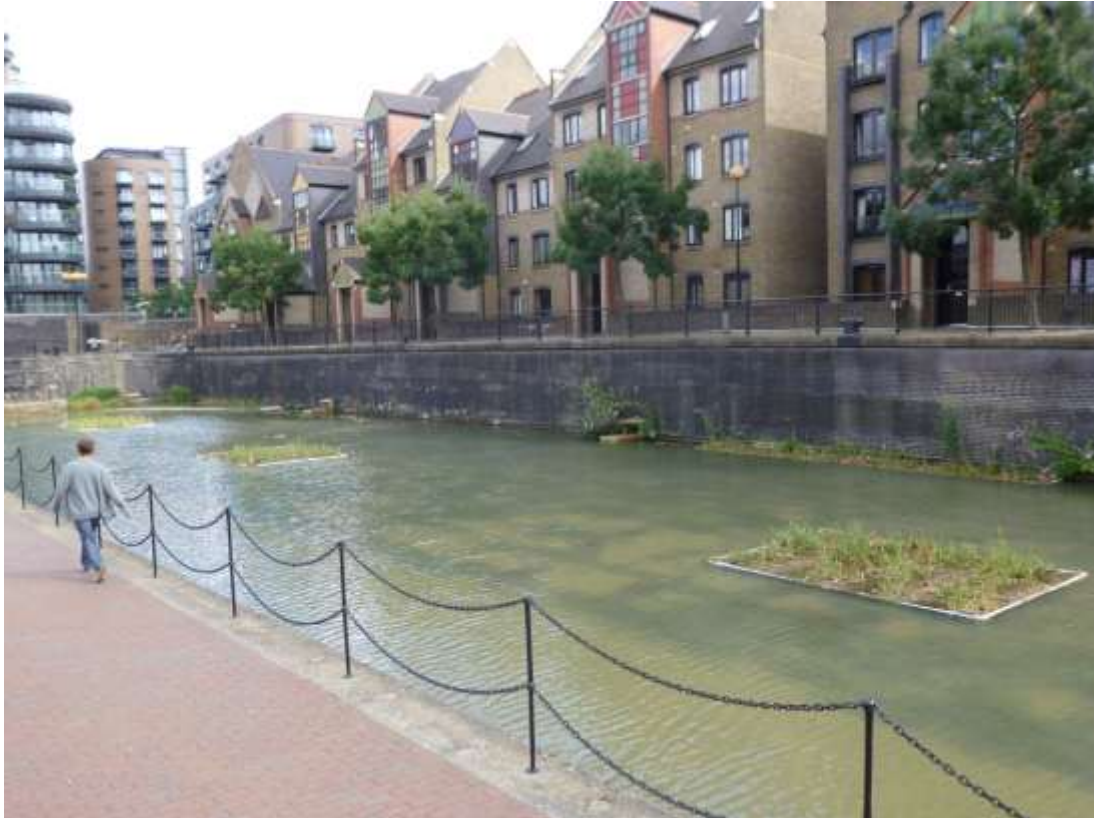
Vegetated rafts in the Wapping Canal (John Archer)
