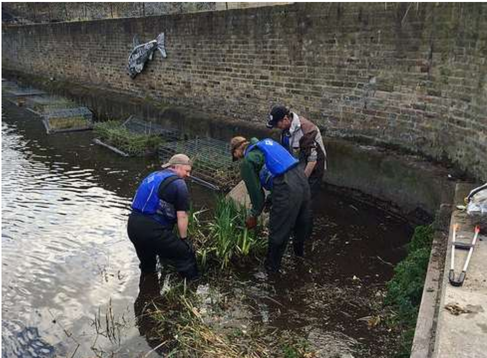
Installing planters in the Regent's Canal (Lower Regents Coalition)
