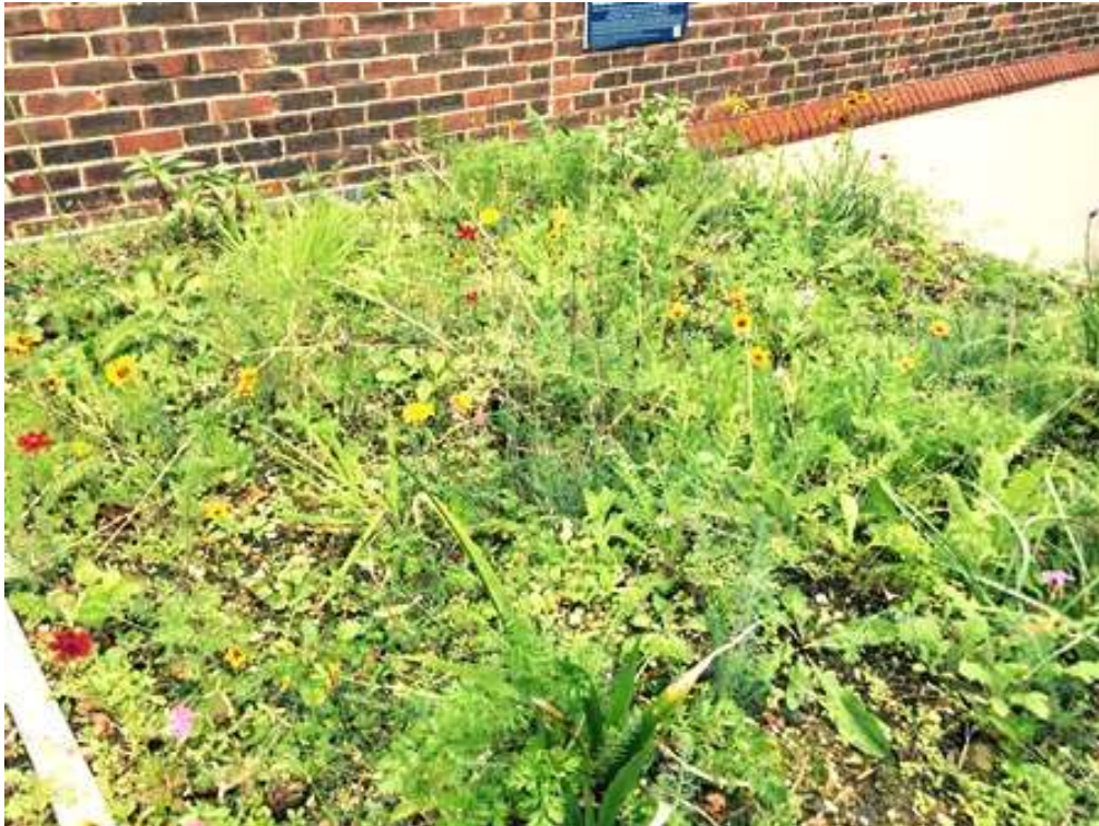
Green roof on cycle store, Westferry Estate (Paul Wilson)
