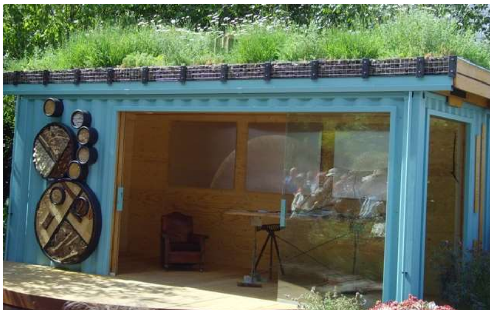
Shed with green roof and bug wall at the 2011 Chelsea Flower Show (John Archer)
