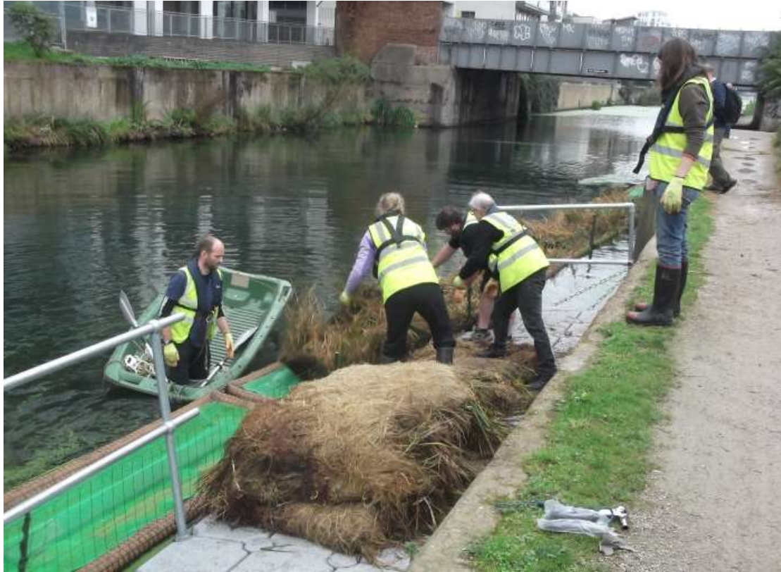
Installing vegetated rafts in the Limehouse Cut (Ben Fenton/Thames21)
