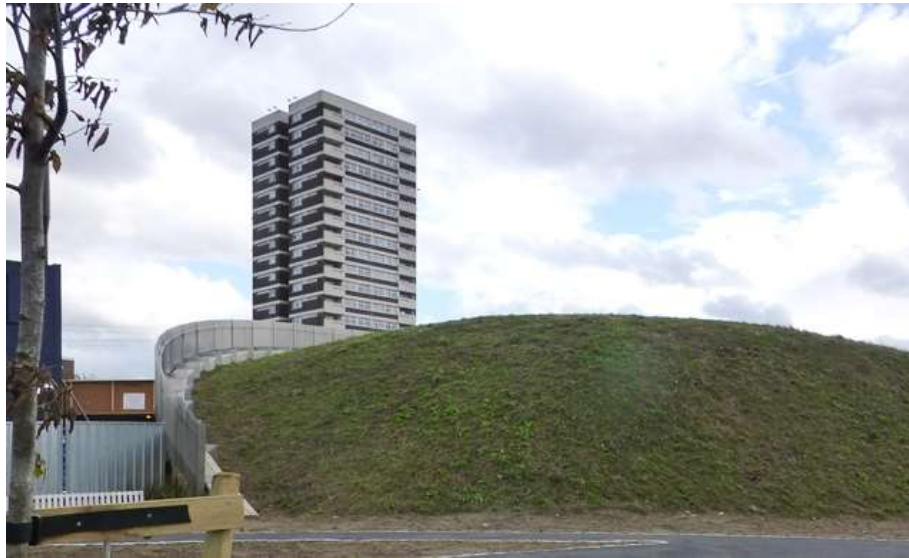
Meadow roof over the Mile End Crossrail vent shaft (John Archer)
