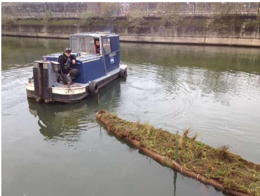
Installing a floating reed bed at Bow Locks (Thames21)
